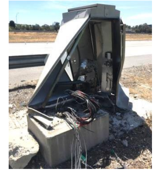
Damaged traffic cabinet from collision along SR-91 Freeway
